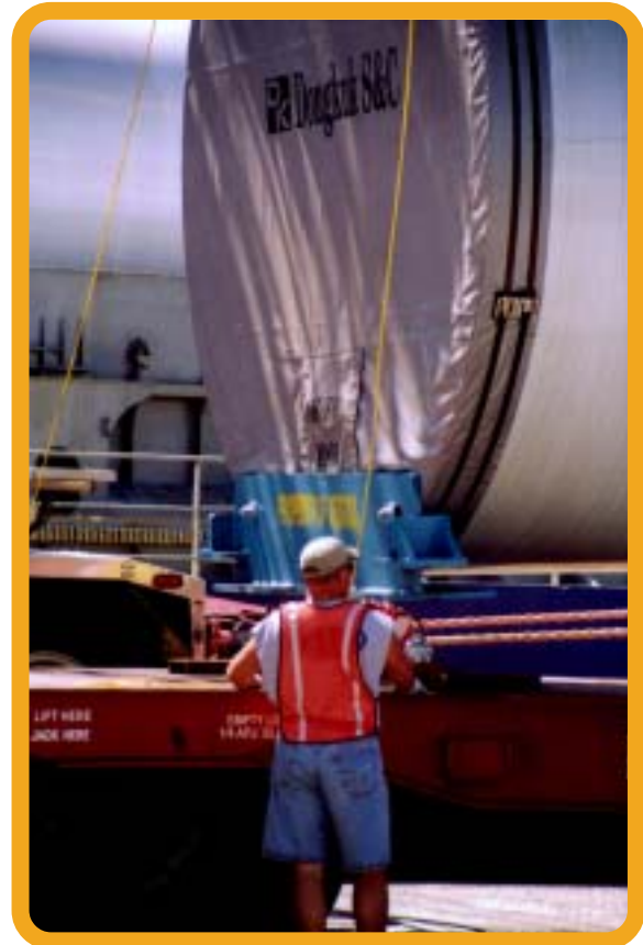
^ A longshore worker secures a 50-ton tower onto an extra-long rail car.
